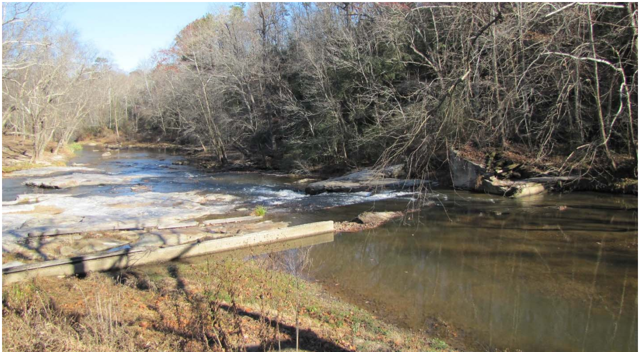
Patterson-Hampton-Sloan Mill Dam remnants, facing east upstream of the mill
