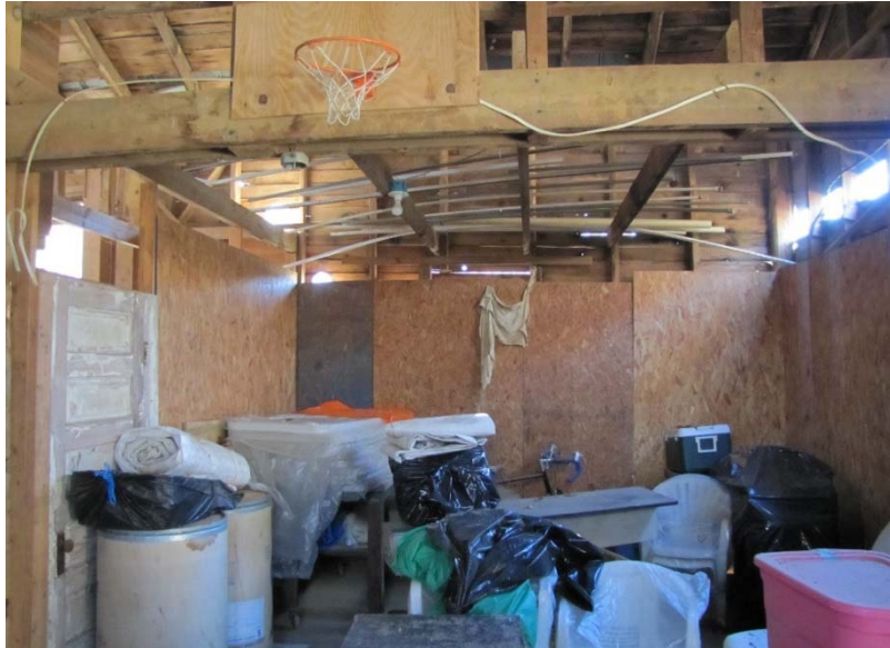
Patterson-Hampton-Sloan Mill, first floor
