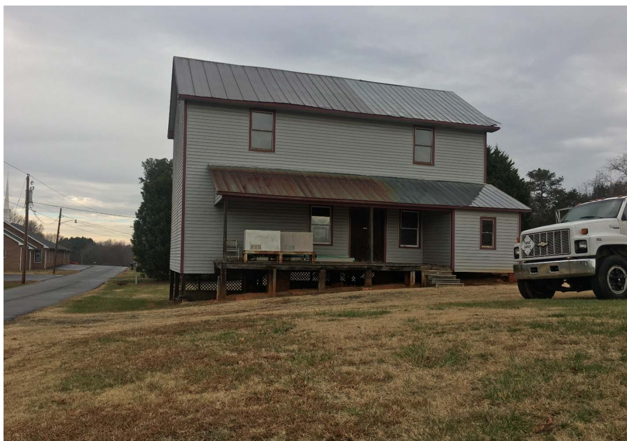
Wilhelm-Smitherman Roller Mill (YD0347). Photos by Author December 2016.
