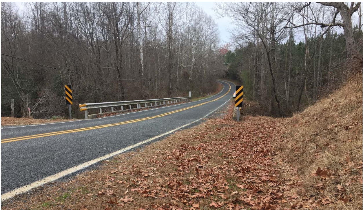
Bridge No. 28 view to the northwest along Sloans Mill Road
