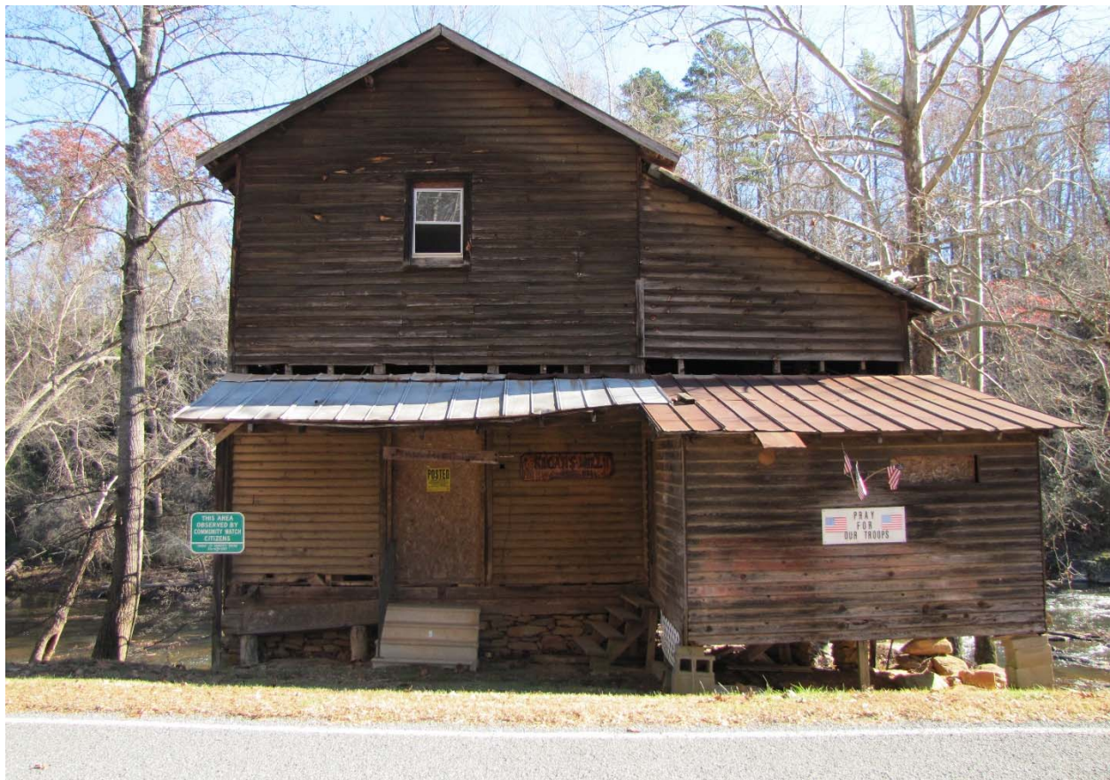
Patterson-Hampton-Sloan Mill (YD 0498), 2712 Sloans Mill Road, façade, view to the east
