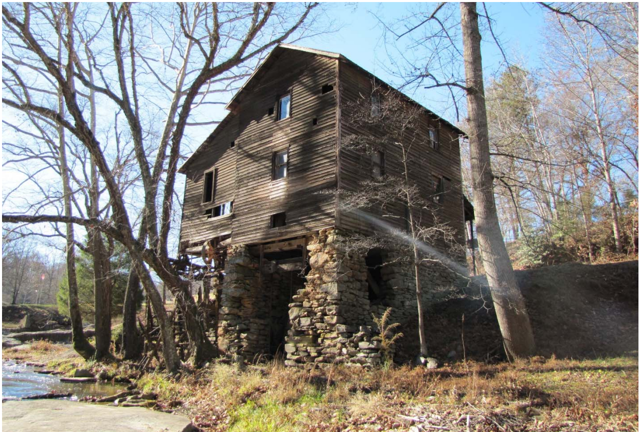
Patterson-Hampton-Sloan Mill, south elevation, view to the west
