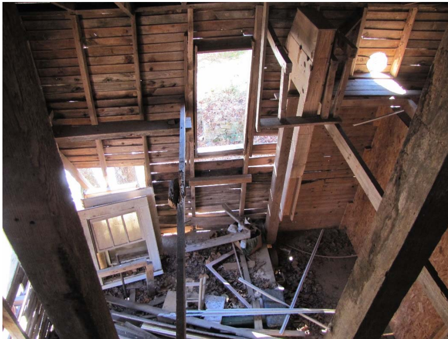
Patterson-Hampton-Sloan Mill, second floor looking down
