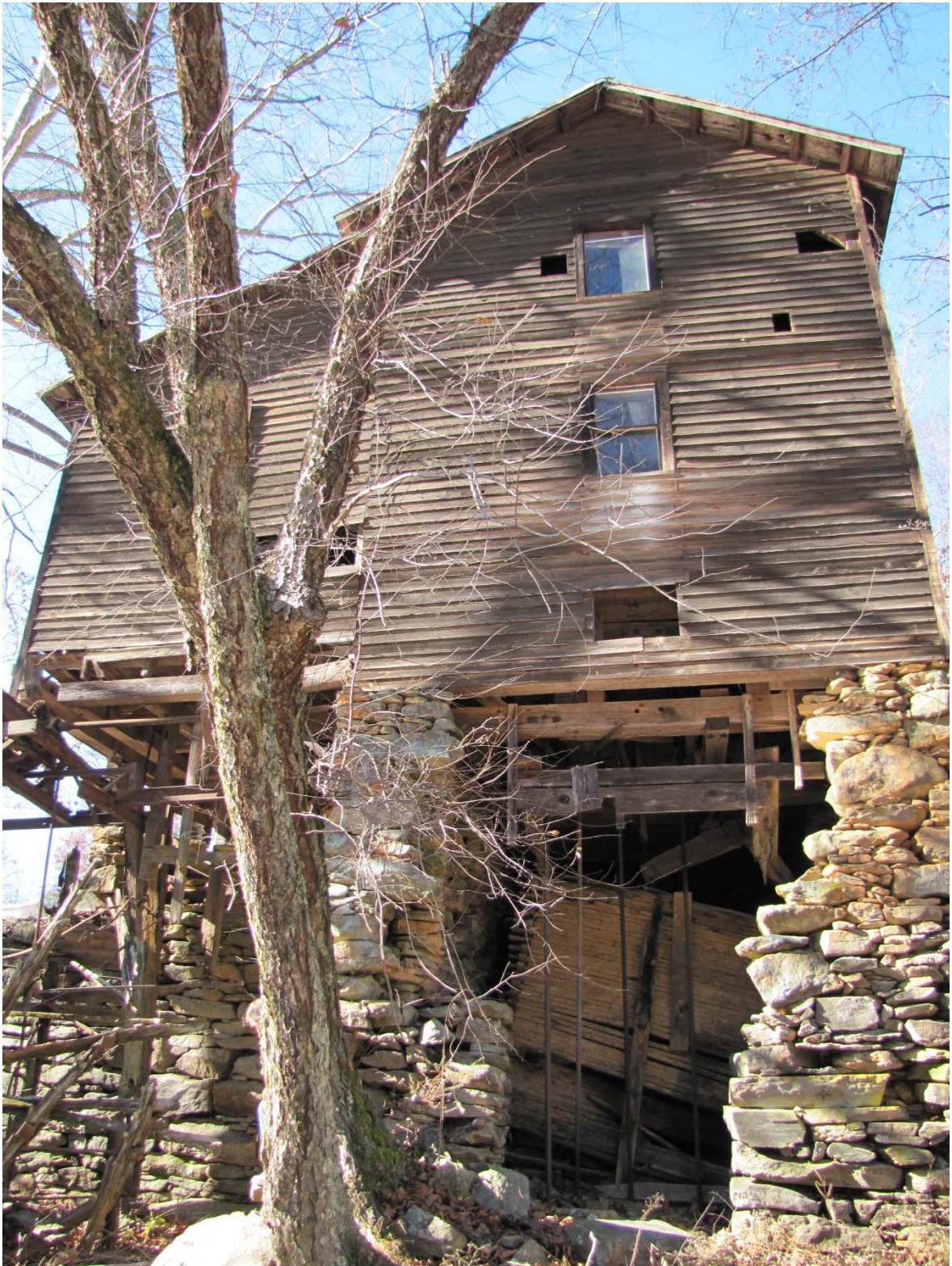
Patterson-Hampton-Sloan Mill, south elevation, view to the northwest.
