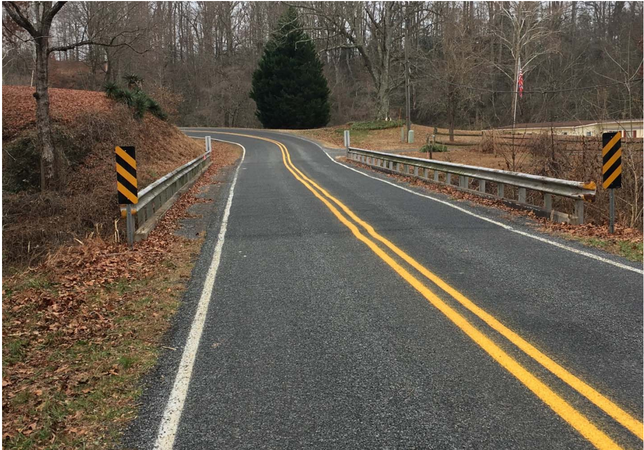
Bridge No. 28, view to southeast along Sloans Mill Road (SR 1119)
