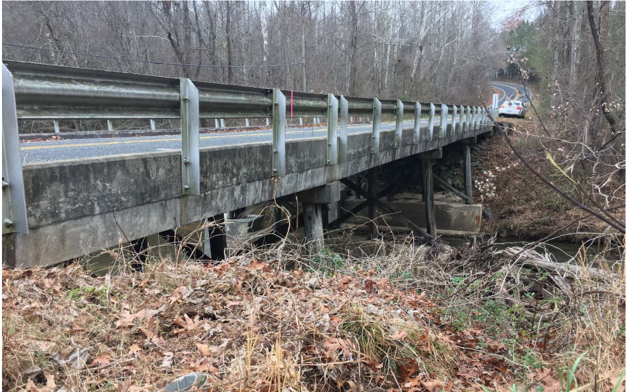
Bridge No. 28, oblique view to the northwest
