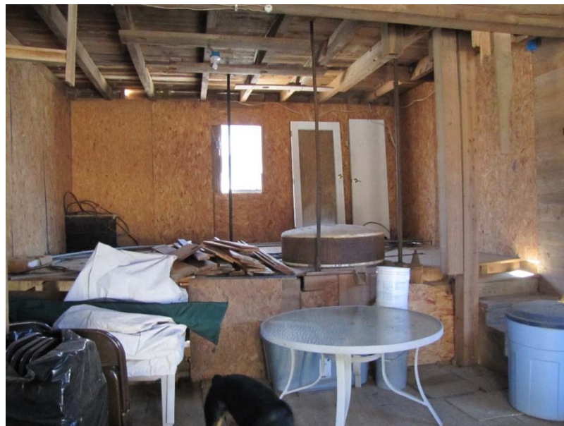
Patterson-Hampton-Sloan Mill, first floor
