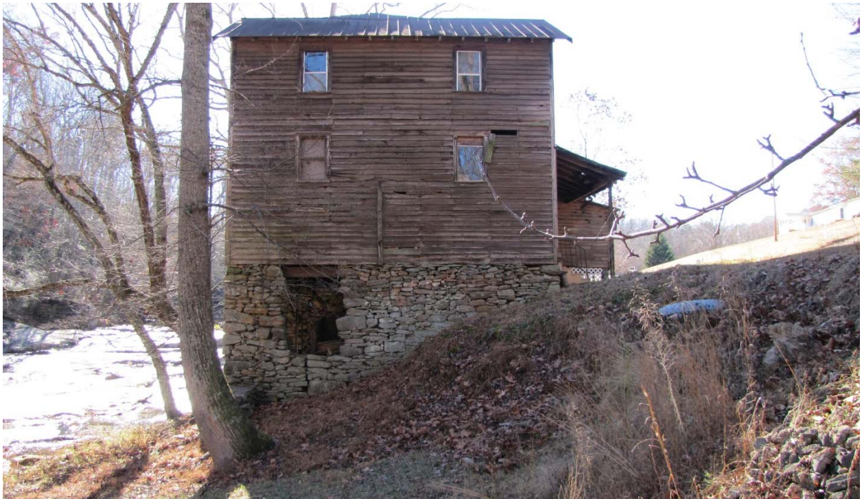
Patterson-Hampton-Sloan Mill, east elevation, view to the southwest
